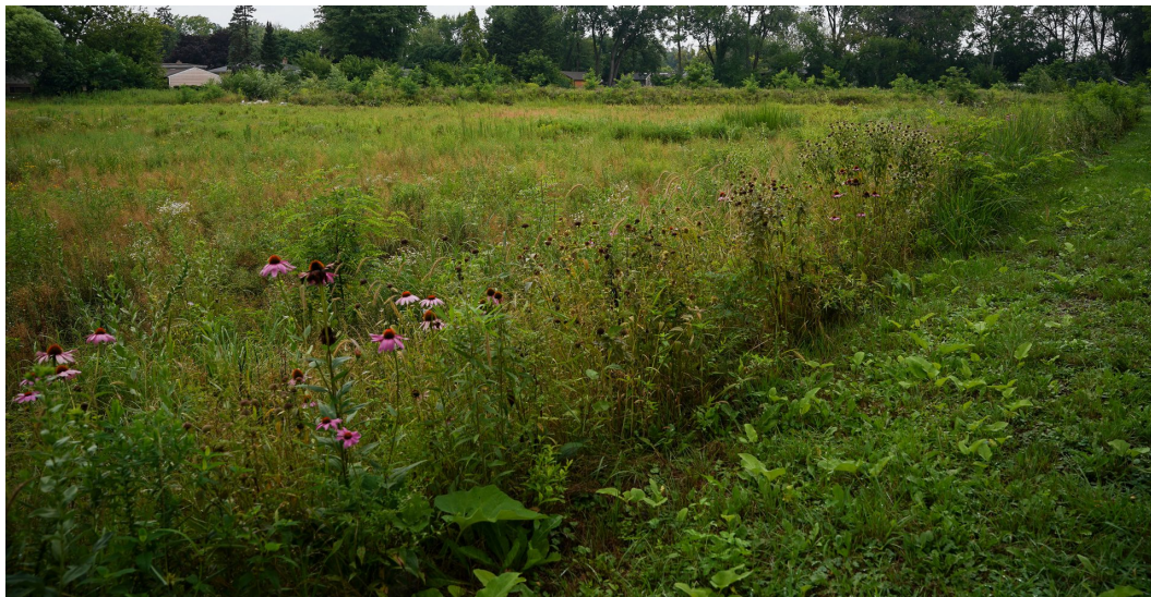
The stormwater storage basin alongside Natalie Creek in Midlothian, Ill., Aug. 5, 2023. During heavy storms, this 1.8-million-gallon detention basin fills up like a pond to mitigate flooding along the creek.
