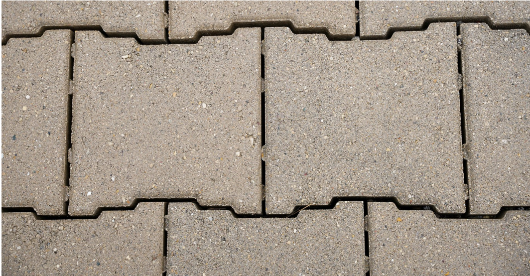
The permeable brick parking lot behind the Veterans of Foreign Wars building allows stormwater to seep through to mitigate flooding in Midlothian, Ill., Aug. 5, 2023.
